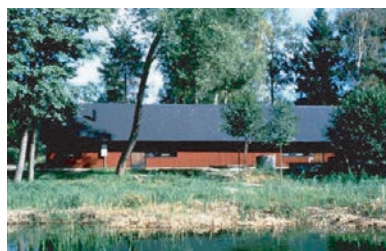
Figure 4.26 Chemical treatment facility at FBM installation at Lake Rönningesjön, Sweden. (Used with permission of Fresh Creek Technologies, Inc.)
