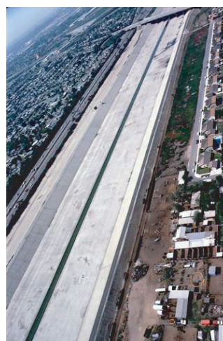
Figure 4.40 Los Angeles River showing small central pilot channel containing perennial flow.
