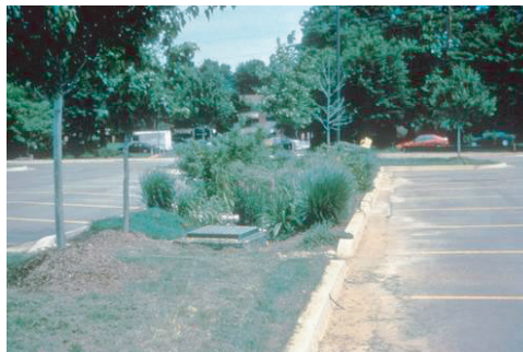
Figure 3.20 Biofiltration in parking area (Photo used with permission of Center for Watershed Protection.)
