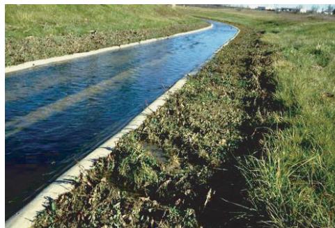
Figure 3.9 Lined channel in Milwaukee, WI.
