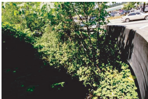
Figure 4.16 Urbanized Kelsey Creek, Bellevue, WA, in commercial area.
