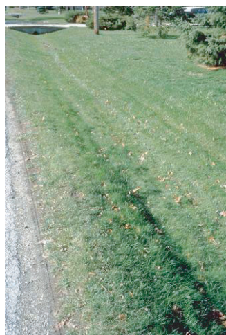
Figure 3.17 Grass swale in residential area, Milwaukee, WI.
