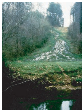
Figure 4.47 Unusual continuous SSO discharge from surcharged/broken sewerage along Five-Mile Creek.
