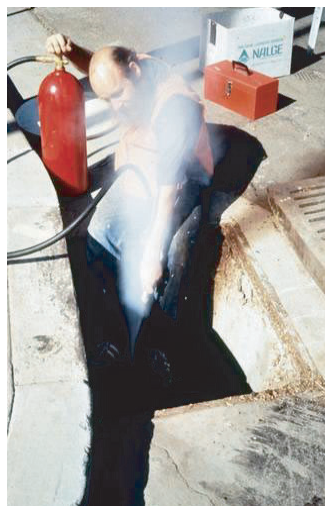
Figure 5.71- Freezing core sampler venting CO 2 used to sample catchbasin sediment in San Jose, CA.
