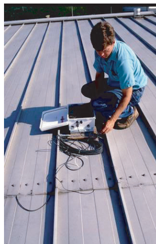
Figure 6.54 Roof temperature data loggers being used by WI DNR.
