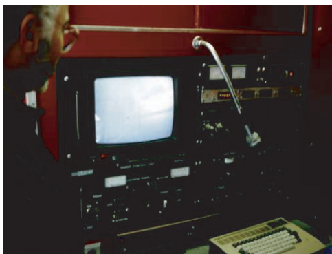
Figure 6.116 Remotely operated TV camera surveys of storm sewers in Boston to locate inappropriate discharges.
