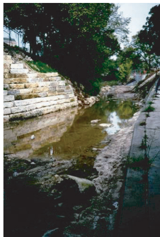
Figure 3.8 Lined embankment along Waller Creek, Austin, TX.
