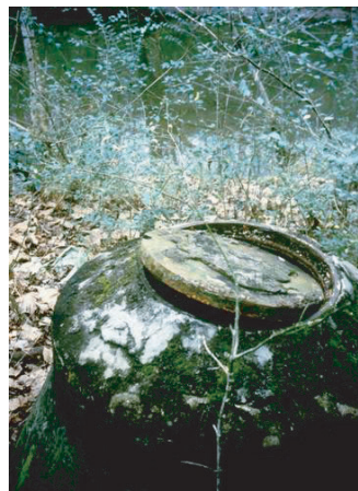
Figure 4.46 Typical SSO discharge point along banks of Five-Mile Creek.
